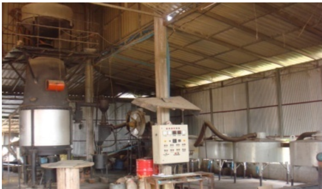
Biomass generator 200 kWe
